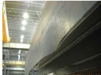
Fig. 9. Mechanical damage of the foot.
