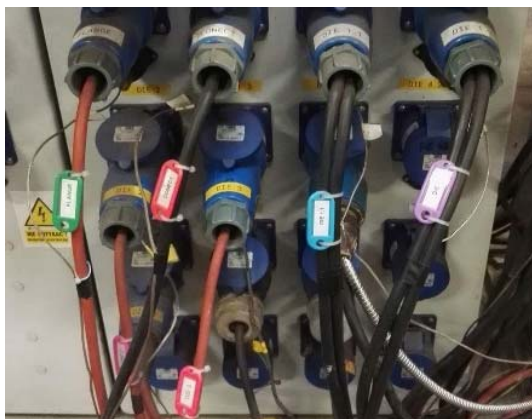
Fig. 3. Corrective actions resulting from the 8D analysis
